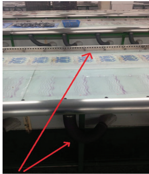
Figure 6 - Downdraft exhaust under adhesive applicator
