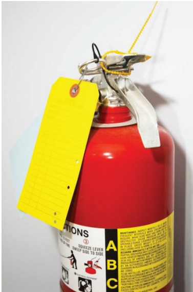
Figure 5 - Fire Extinguisher with Inspection Log.
